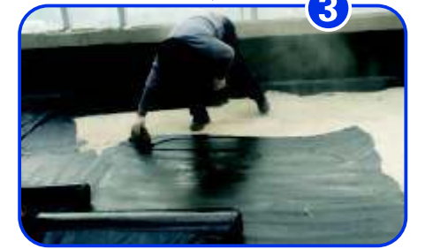
Brush the rubber bitumen waterproof coating
