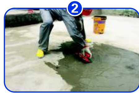
Brush cement mortar
