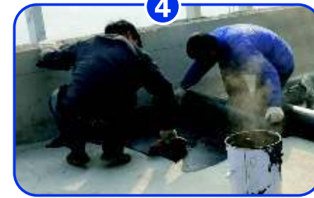
Pave and paste waterproof membrane
