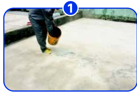
Substrate clean and wet
