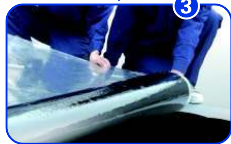
Pave waterproof membrane
