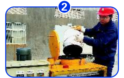
Heat the rubber bitumen waterproof coating
