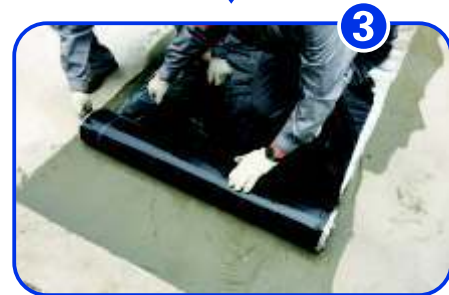
Pave the waterproof membrane
